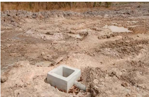
Small earth dam at Kpenayiri in the Bole Bamboi Constituency, Savannah Region
