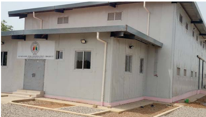
1000 Metric Tonne Grain Warehouse, the Ejura, Ejura-Sekyeredumasi Municipality, Ashanti Region
